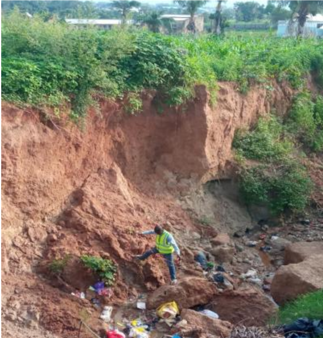
Plate v: Gully Erosion Site at Kuchiyako Ext. III, Kuje.
